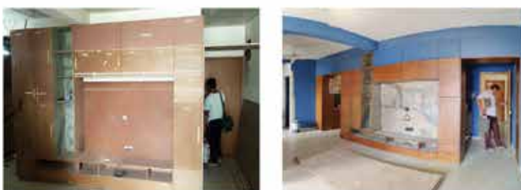
Process Site photos
